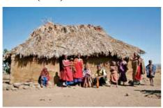
The huts (engaji) of the Maasai are constructed from dried cow's dung, loam soil and hundreds of wooden branches. In the huts, in which small animals also sleep, there constantly burns a small fire which, during the day serves for the cooking and which, in the evening, keeps away mosquitoes and provides
